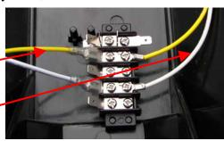
For Flasher and Stop Alert cabinets: pass-through wiring connectors are located inside the Flasher Controller cabinet..
