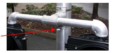
Use a conduit hole plug when wiring through the pole.
